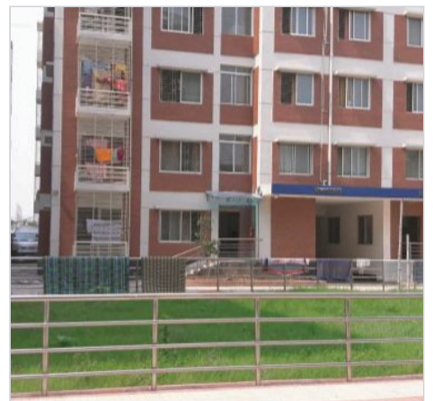
BEPZA Officers Quarters Dhaly Construction Ltd. · Uttara, Dhaka
