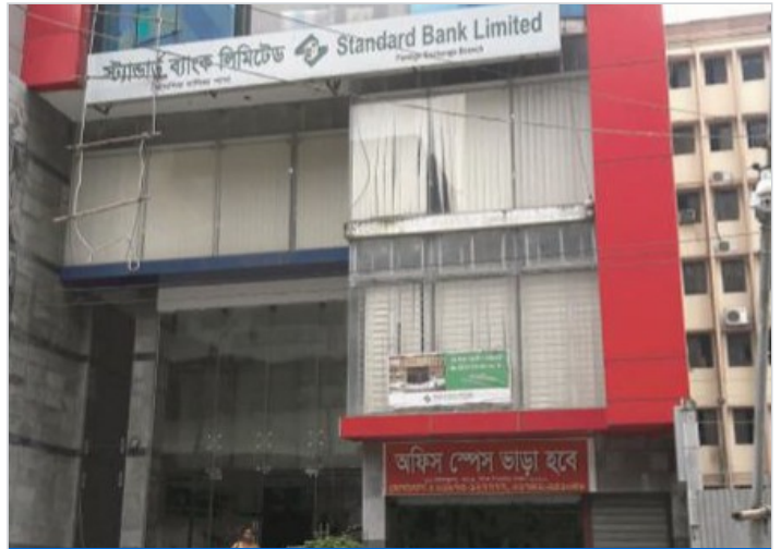
NIC Tower — Curtain Wall Bishal Builders · Dilkusha, Dhaka
