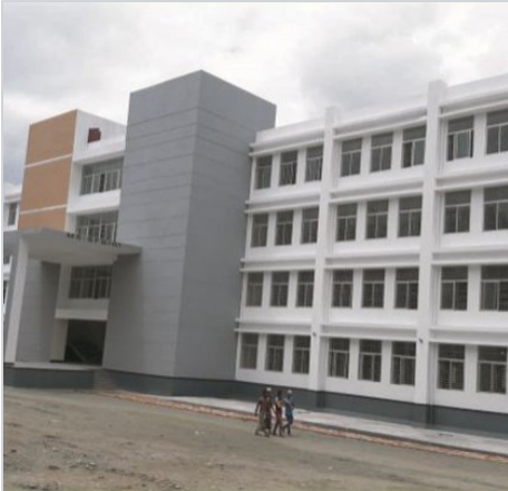
Adamjee EPZ Modern Factory 1-3 Hossain Construction · Adamjee EPZ
