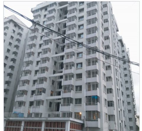
Ansar Camp Housing Project Jewel Construction · Mirpur, Dhaka
