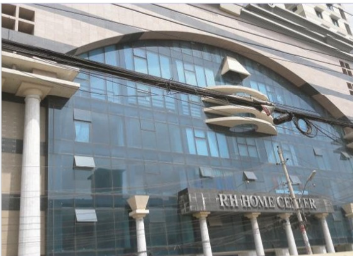
RH Home Center — Facade & Glass Work KS Engineering · Green Road, Dhaka
