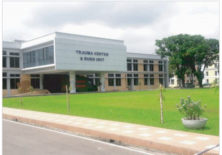
Trauma Center & Burn Unit, CMH Hossain Construction (Pvt.) Ltd. · Dhaka Cantonment
